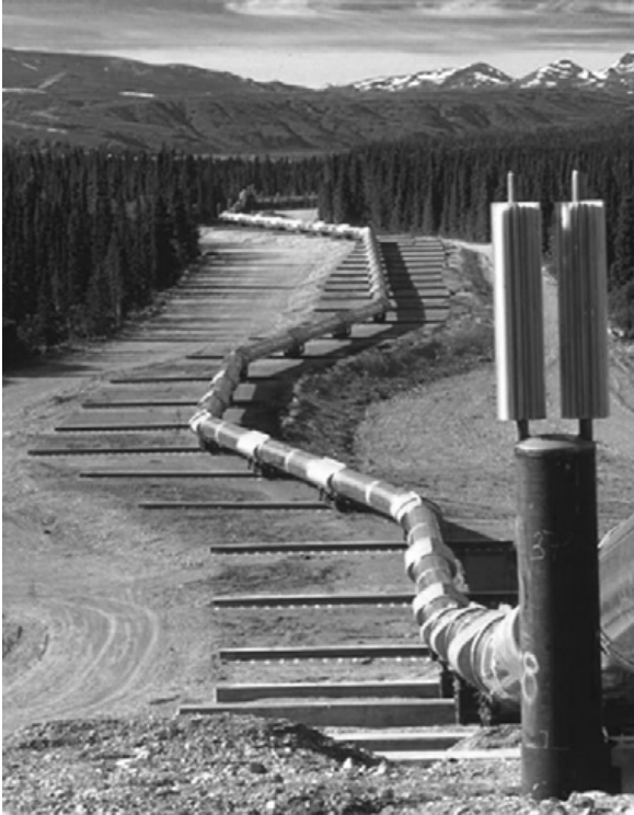
Figure 2 – Original pre-earthquake alignment view of Denali Fault crossing, looking south
