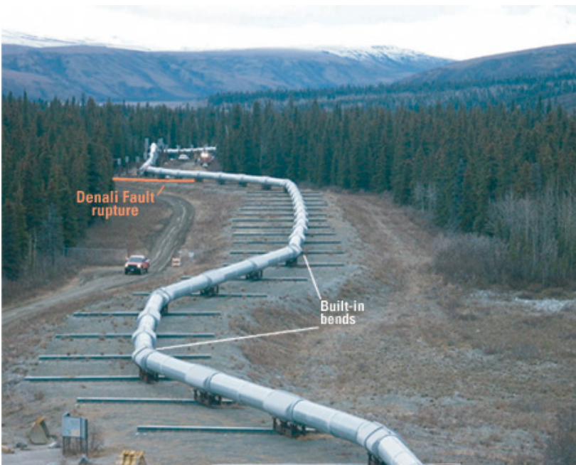
Figure 3 – Post-earthquake alignment from similar vantage point, looking south, showing compression bending and displacement
